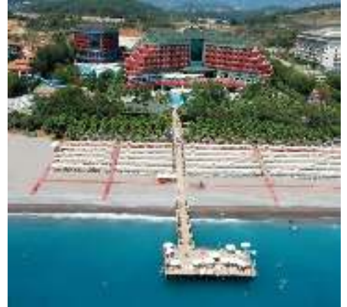
Main Building and Annex Building
